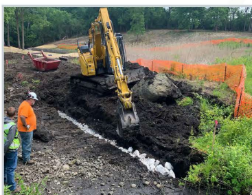
Stone toe installation
