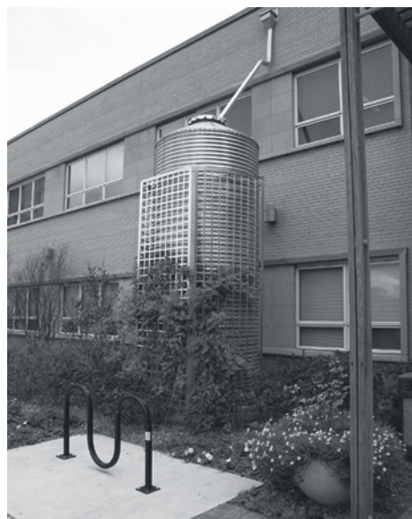
Rain barrels, such as this one in Chicago, capture roof runoff for other uses.
