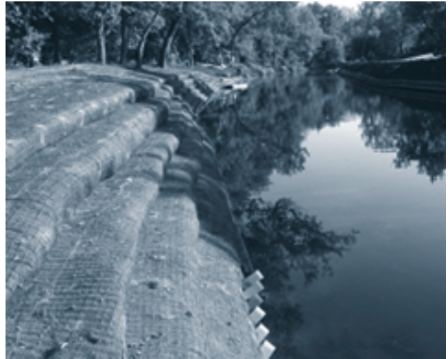
Streambank stabilization using bioengineering methods.
