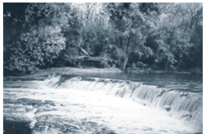
A low-head dam on Salt Creek.
