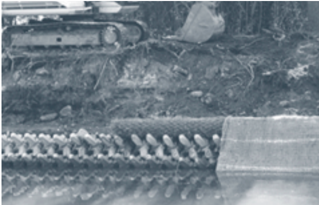
Stabilization using A-Jacks, fiber rolls, and erosion control matting.
