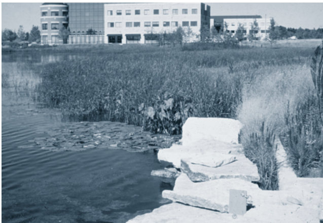
Natural detention basin at Prairie Stone business park in Hoffman Estates.
