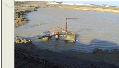
Dewatering...Floating the Pump
