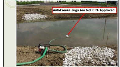
Dewatering...Floating the Pump
