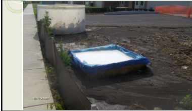
Construction Washout
